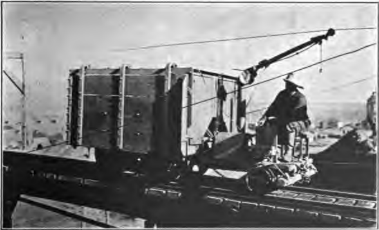
THREE-TON TRAM CAR WITH MOTOR USED ON ONE-LEG TRESTLE.—COLBY MINE
